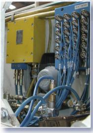
Dual power supply unit dNTA42 for the supply of voltage to an electrohydraulic control unit
